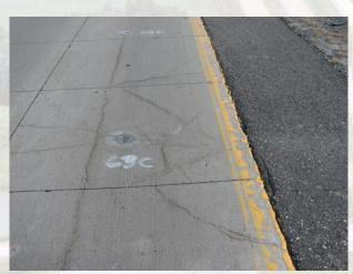
Figure 3. Cracked and "shattered" panels in Cell 63 (Fall 2010).
