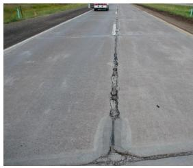
Figure 3.4. Typical Transverse and Longitudinal Joint Condition Prior to Overlay
