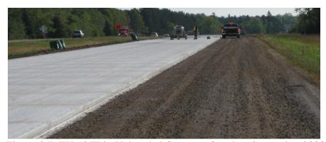
Figure 3.7. TH 53 Thin Unbonded Concrete Overlay, September 2008
