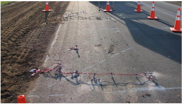
Figure 2.4. Installed Instrumentation Prior to Paving the Overlay [September 9, 2008]
