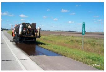
Figure B.7. Starting to apply fog seal
