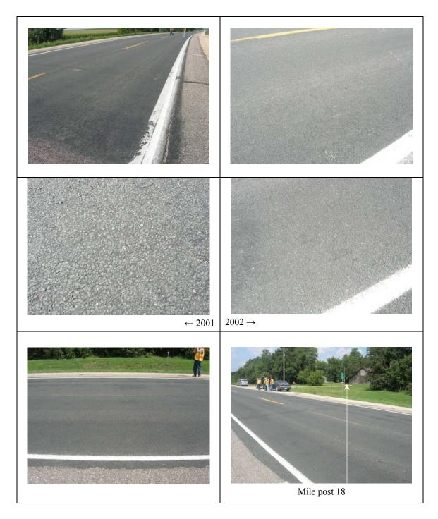
Figure C.6. TH 56 sections with surface treatment applied in 2001 and 2002 (built in 1995), mile 16 to 17 and 17 to 18, respectively
