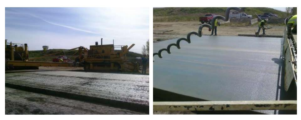
The lower lift comprised of recycled concrete as the source of coarse aggregate. The upper lift used the high quality, Class A aggregates.
