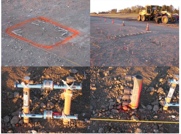
Figure 4. Instrumentation installed prior to placement of the PCC to measure pavement responses to temperature and traffic loads (dynamic strain gages – top left, static strain gages – bottom left, humidity sensors – bottom right, overall view – top right)
