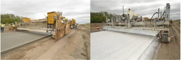
Figure 5. Texturing and curing of the RCA PCC
