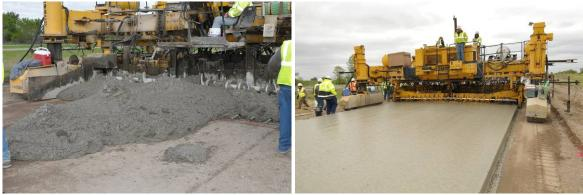
Figure 3. Placement of the RCA PCC layer
