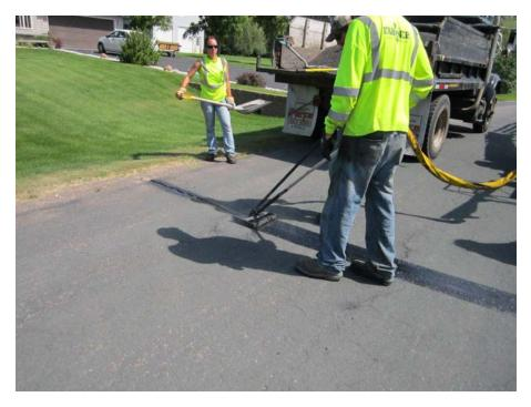
Figure 8 – Cover aggregate awaiting sealant and squeegee installation
