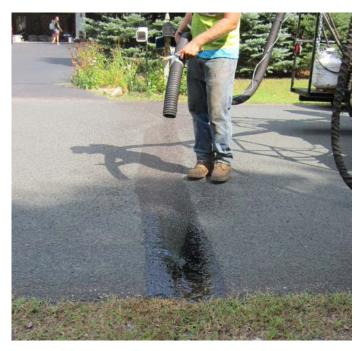
Figure 21– 1<sup>st</sup> pass with cover aggregate
