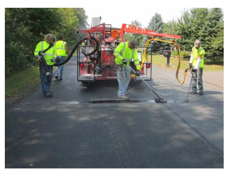
Figure 9 – Typical Operations, Mechanical Aggregate placement, Squeegee & Sealant Wand
