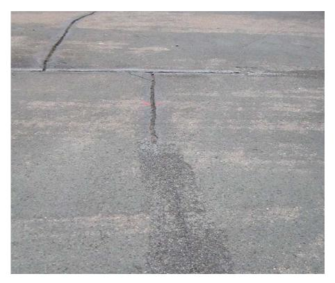
Figure 15 – Clean & Seal ½ completed – Note 3/4+ crack size
