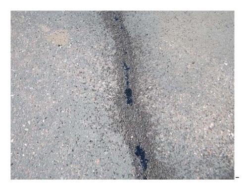
Figure 6 – Bleeding of Flush Filled, Routed Crack – Typical of Shoved Cast Rock
