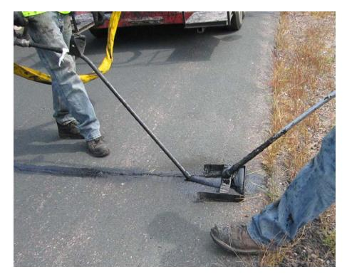
Figure 7 – Typical filling of squeegee for leveling operations (1ft. squeegee pictured)
