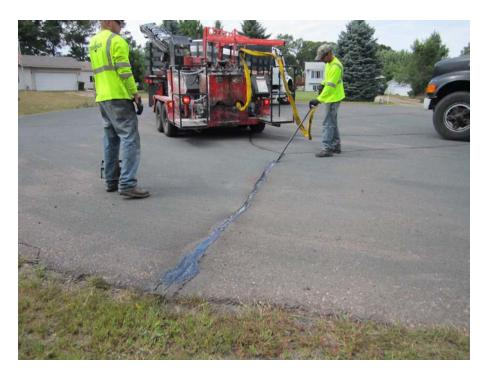
Figure 5 – Flush Filling of Routed Crack
