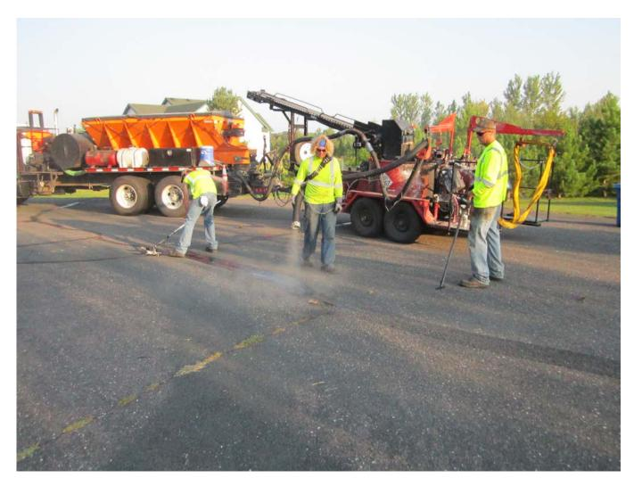
Figure 16 – Squeegee, Wand and Mechanical Aggregate mobility from trailer
