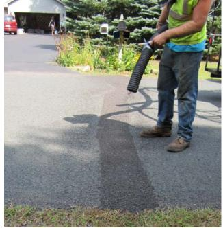
Figure 22 – Finishing with extra cover aggregate
