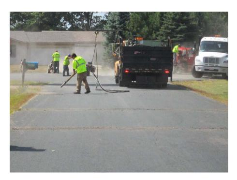
Figure 4 – Routing, Cleaning and Heat Lancing of Cul-de-sac
