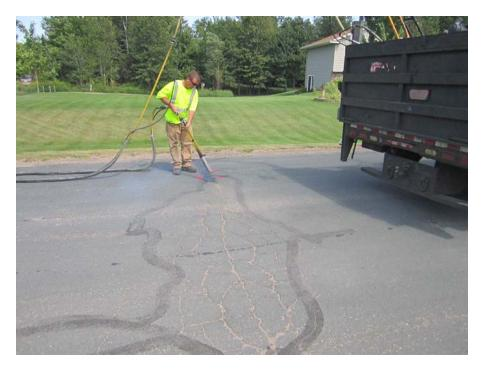
Figure 1 – Heat Lance operations before sealing – Typical for all operations
