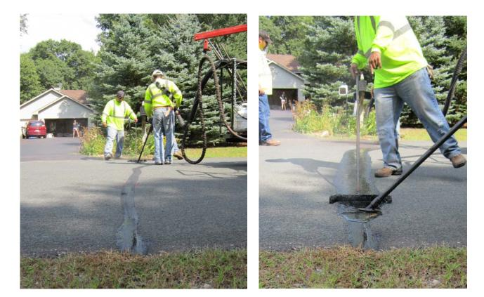
Figure 19 – To be repaired crack, heat lanced
