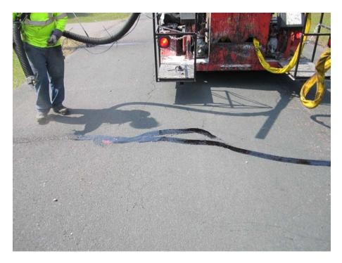
Figure 14 – Clean & Seal Repair area
