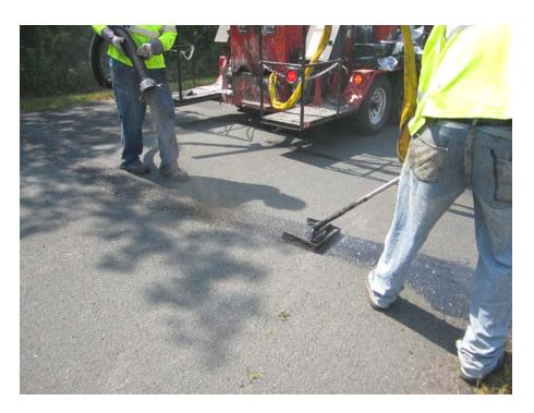
Figure 10 – Leveling and placement operations
