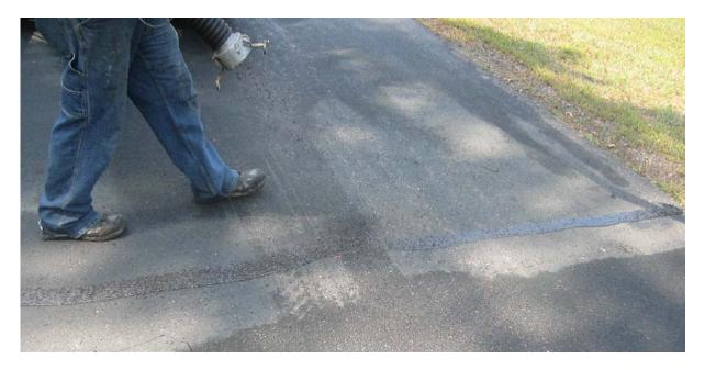
Figure 11 – Finished 3in. Squeegee with cover aggregate
