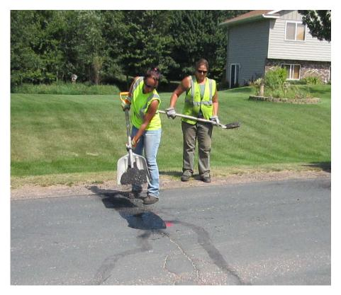
Figure 3 – Shovel Casting of Cover Aggregate
