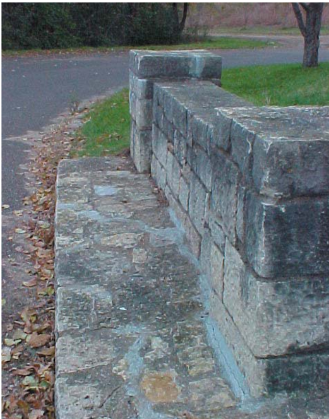
Wall / Walk termination at southwest
