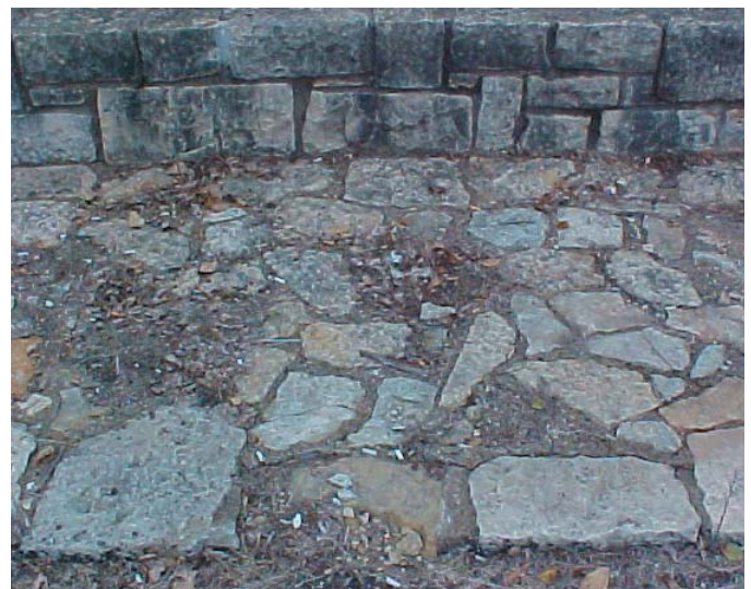
Typical flagstone condition
