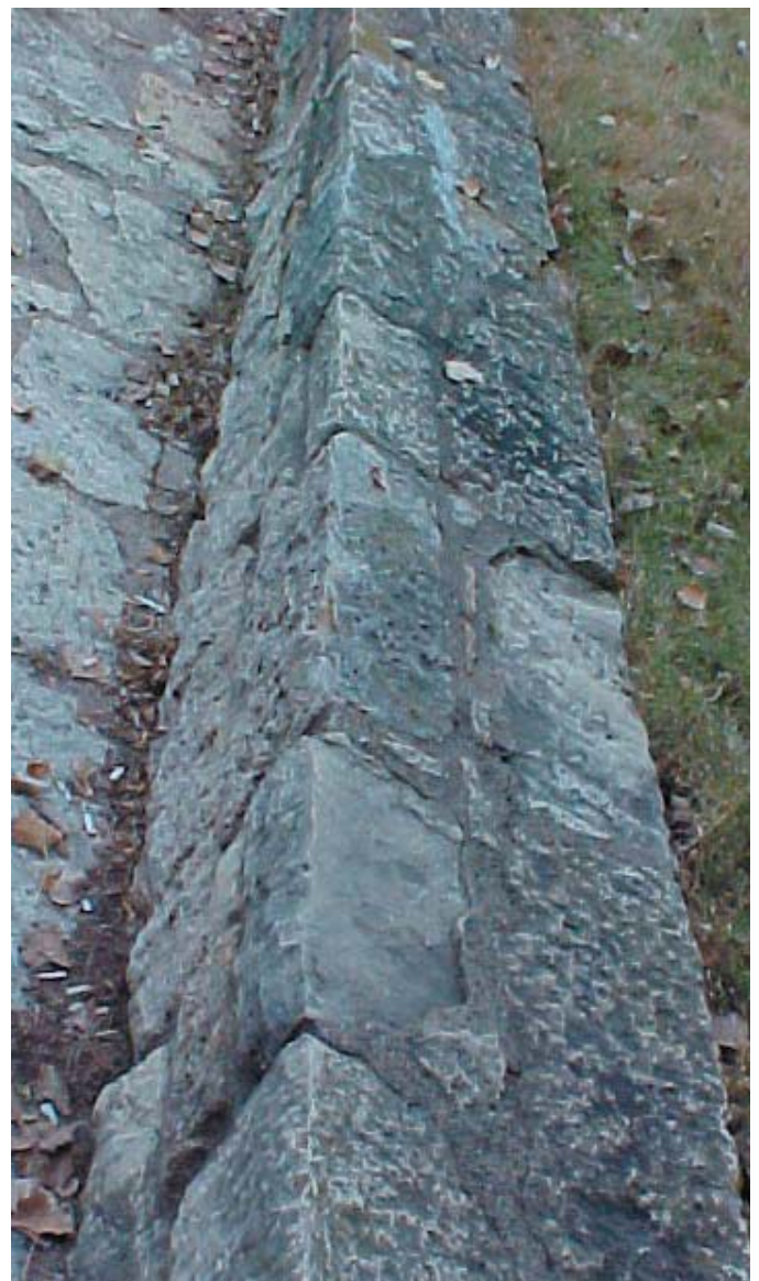
West wall condition
