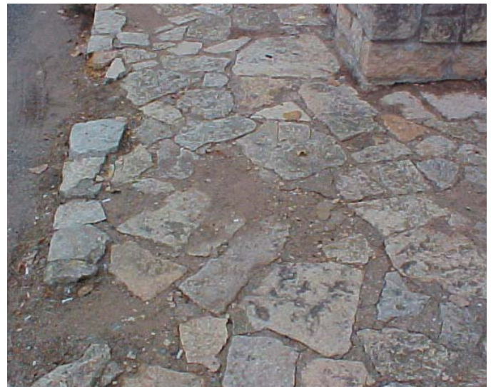
Flagstone condition at northwest (near pedestrian entrance)
