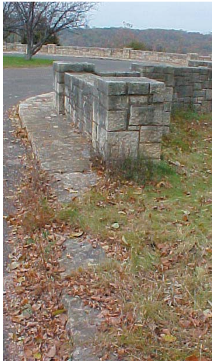
Wall / Walk termination at southeast
