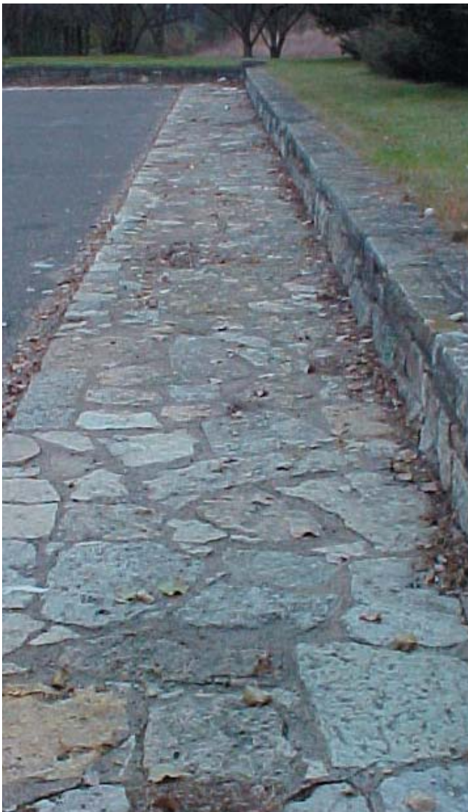
Flagstone walk condition at west end - looking north
