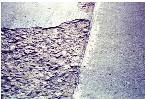
FIGURE 27: CONCRETE PAVEMENT PATCHING
