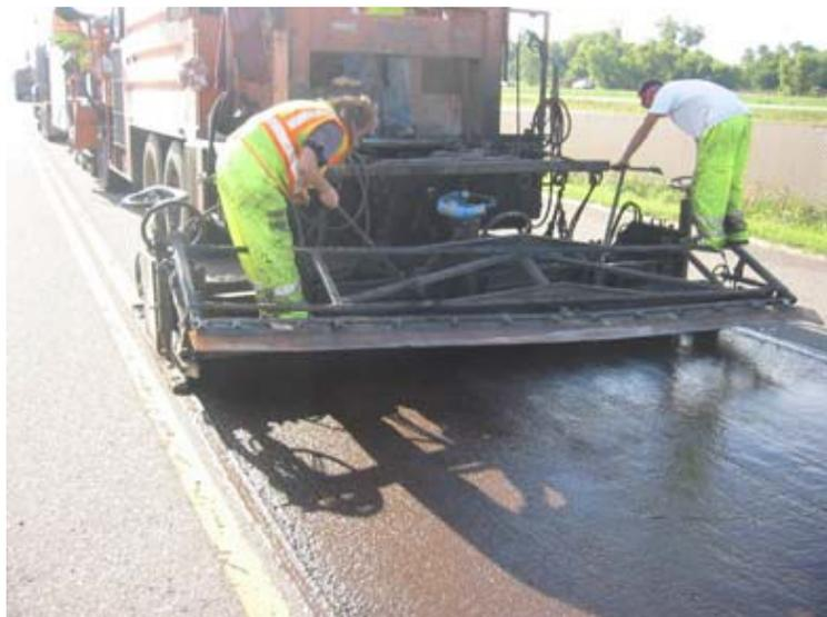
A distressed asphalt pavement requiring a surface treatment such as microsurfacing is shown in [Figure 6](#). A typical microsurfacing operation is shown in [Figure 7](#).
