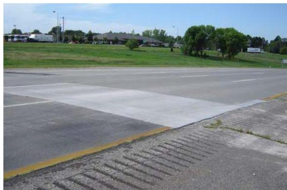
of new supporting base materials, and compaction of these materials backfilling with proven asphalt materials. High early strength concrete may also be used on roadways with high traffic to obtain quick re-opening to traffic. Even newer technology using pre-cast and reinforced concrete slabs inserted into the previously prepared blow-up area may be used to obtain quick re-opening of traffic.
