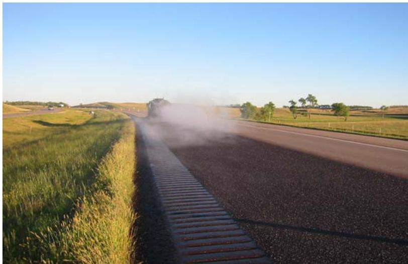
as pavement friction (skid resistance) may be reduced until some of the asphalt material is worn off. Information on application techniques and material rates can be found in the [Minnesota Seal Coat Handbook 2006](#), the MnDOT [Best Practices Handbook for Asphalt Pavement Maintenance](#), and the [MnDOT Distress Identification Manual](#). Fog sealing of a road shoulder is illustrated in [Figure 3](#).
