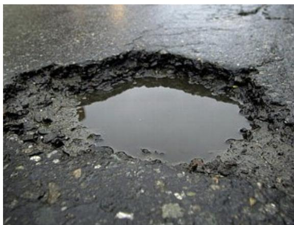
Semi-permanent patching involves more pothole preparation prior to placing the patching material. The pothole may be cleaned with air and debris removed but not saw cut. Permanent patching is used when the pavement is still in good condition, traffic control can be provided and needed resources are available.
