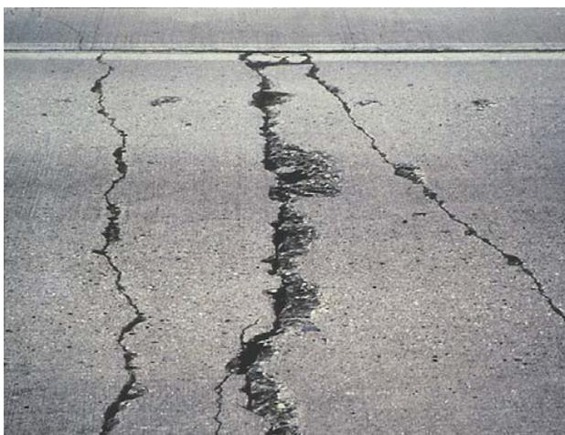
FIGURE 21: LONGITUDINAL RANDOM CRACKS IN PCC PAVEMENT
