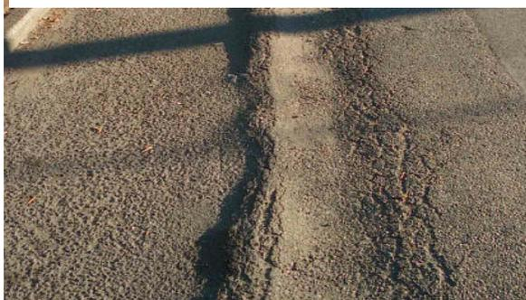
[Figure 11](#). Microsurfacing with a slurry mix or use of mastic material could be considered an alternative to tight blading (see [Section 3-4.04.01.05](#) above for information on microsurfacing).
