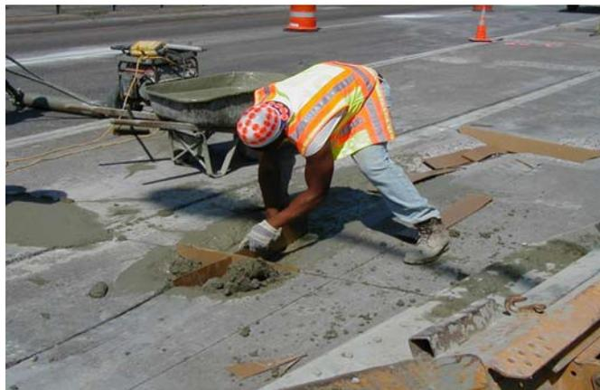
Concrete mixture for patching larger distressed areas should adhere to the following:
