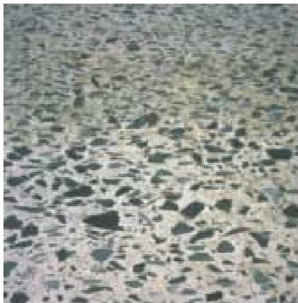
FIGURE 26: SCALING OF CONCRETE SURFACE
