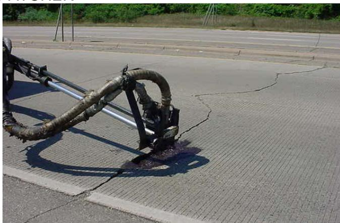
Patching may also be done using a spray injection technique (“blow patching”) where air pressure is used to apply a mix of fine aggregate and asphalt emulsion into potholes or large cracks. Still another effective patching technique involves the use of mastics which are a proprietary blend of asphalt sealants and aggregate. Specifications for patching materials and procedures are covered in MnDOT specifications and special provisions available from [MnDOT Materials Engineering](#). An
