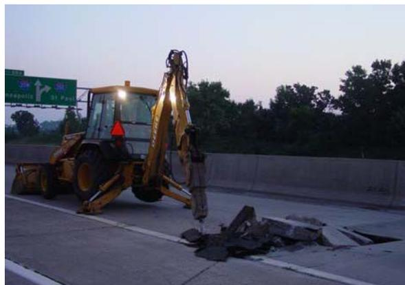
FIGURE 17: BLOW-UP REPAIR
