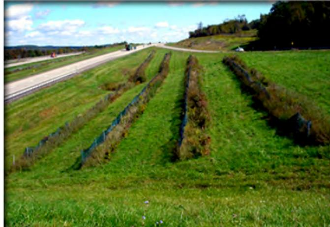
**Project Description:** Keeping snow and ice off of windswept areas of the roadway can be aided by the installation of a traditional snow fence, tree and shrub planting, and by leaving standing corn rows in farm fields. In roadway ditch rights of way where these methods are not an option or have proved to be too expensive to implement, the district will plant a 10-foot-wide swath of tall native grasses and a 5-foot-wide strip of a perennial cone wildflower mix to serve as a windbreak.
