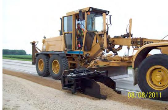
**Project Description:** The district built a wedger to attach to its motor grader to provide greater flexibility in repairing shoulders. Mounting the wedger on the blade of the motor grader allows the blade to slide left and right to do the shouldering work that is typically performed by a shouldering machine. The grader stays on the mainline pavement while the wedger smooths the shoulder.
